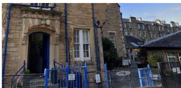
19 - Cathcart Place Entrance (Main Door and Office)
